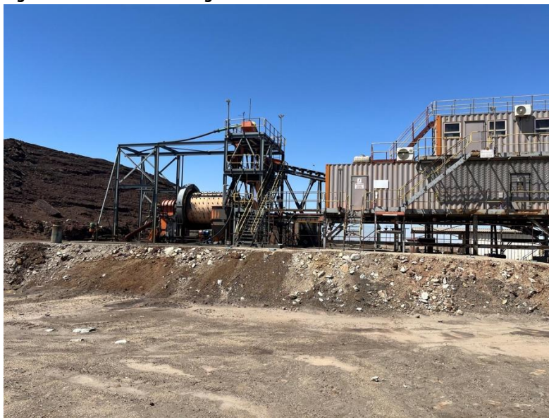
Figure 18A: NLZM Processing Plant: Mill and associated infrastructure
