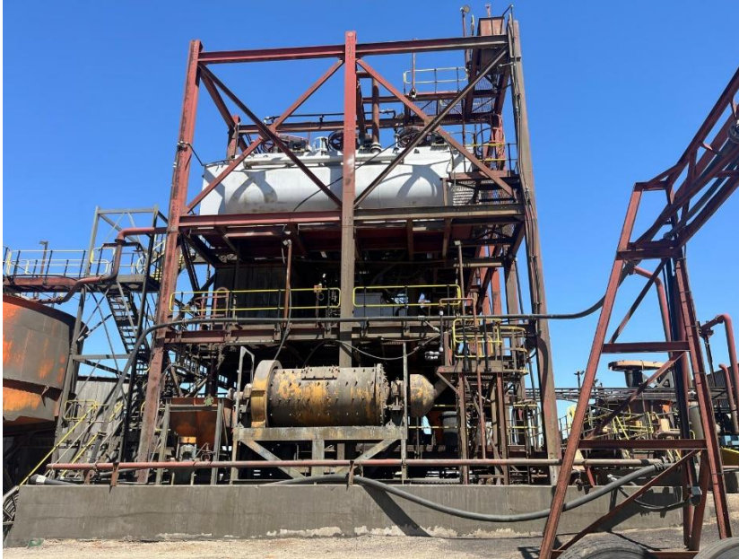
Figure 18D : NLZM Processing Plant: Flotation
